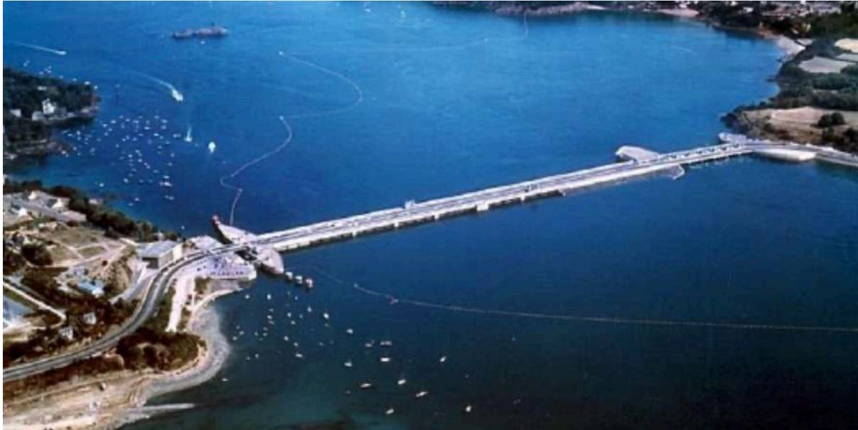
*The Rance Barrage. The access lock is to the left, the generators to the right*
